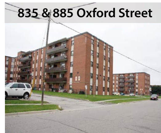
Five storey twin apartment buildings with balconies and four elevators; ≈220 surface parking stalls surround the properties.
