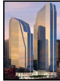
Eighth Avenue Place – East and West
