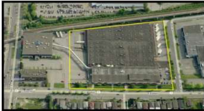
Aerial Photo of the Property
